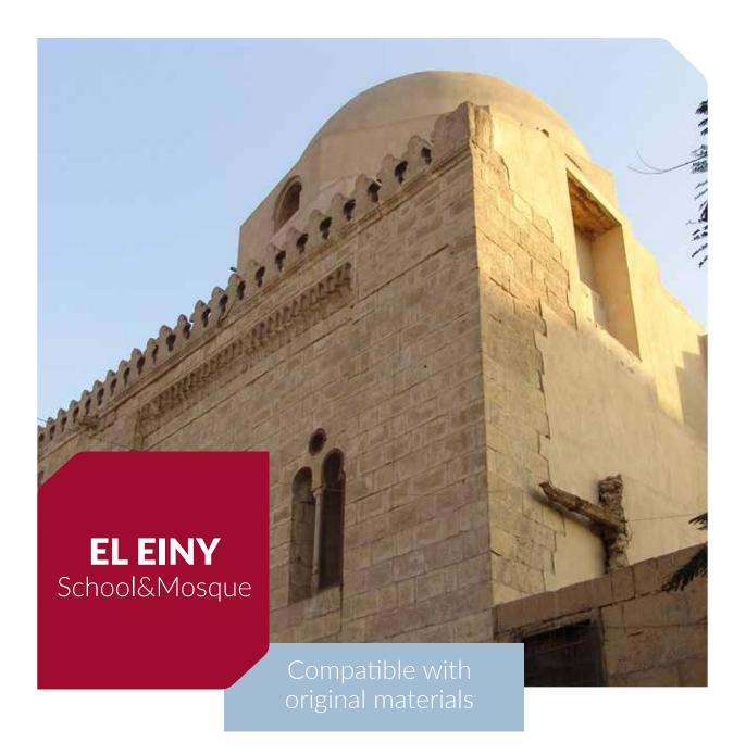
Contently, RME took responsibility for repairing such historical building which required restoration works from several aspects. Among such works, RME was required to protect this establishment and prevent its collapse by injecting its walls with new mortar, which RME carefully selected to be compatible with the original materials
