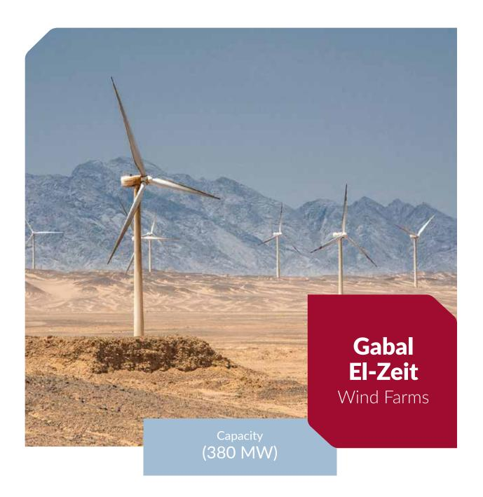
RME was responsible for complete civil works for the 190 Wind Turbine Generator (WTG) footings and WTG platforms. Scope also included the complete network of new internal roads leading to every wind turbine position.
