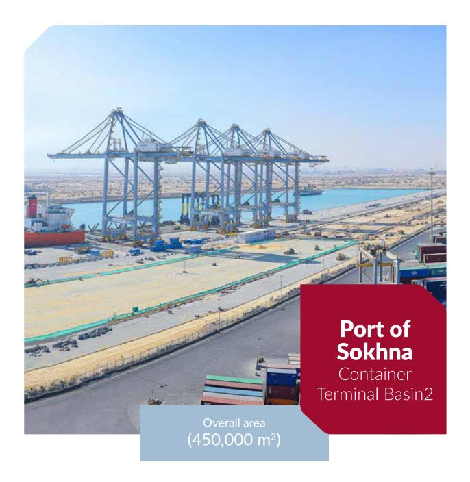
Turnkey construction of a 150,000DWT class new multi-purpose terminal with length of 500 m to satisfy the throughout forecast of 1.75million TEU Containers as well as General Cargo. The Overall area of the terminal is 450,000m². The maximum daily occupancy for the port is 2000 persons.
