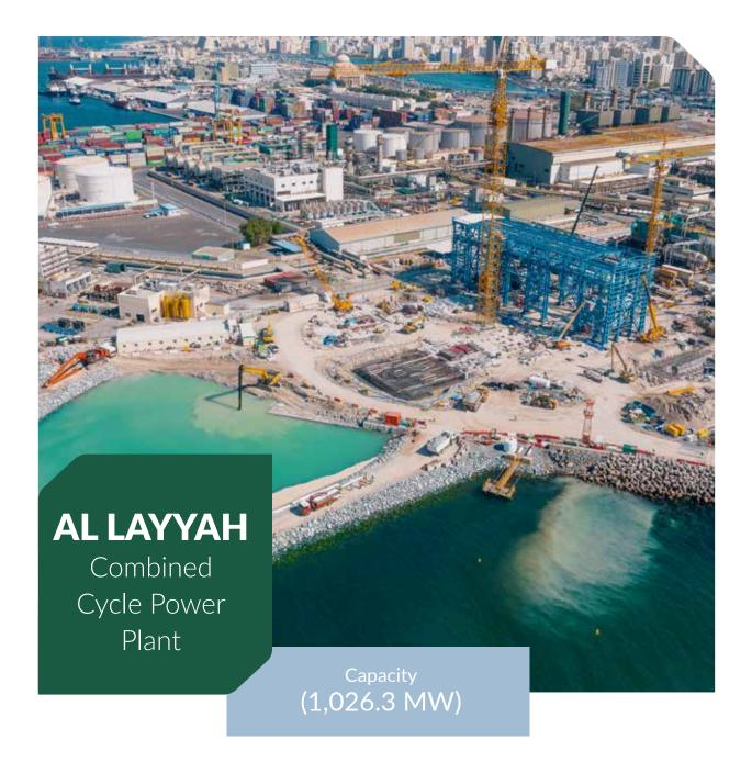
The 1,026.3-megawatt gas-fired combined cycle power project is located in Al Layyah in the Emirate of Sharjah and shall start producing energy by 2020. The power plant will consist of one power block manufactured by MHPS contains two M701F gas turbines, two heat recovery steam generators, one steam turbine, and three generators.
