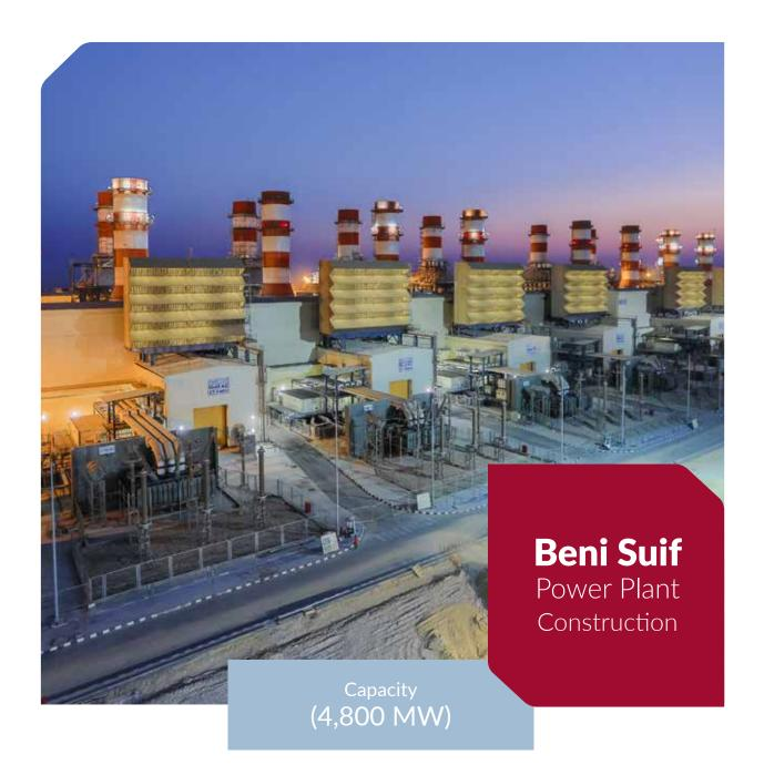
RME was responsible for all the Site Preparation, Execution of all civil, Structure, architectural, and MEP building services for, GIS Area, modules 4 & 3, Gas Turbines 42 ,41 ,32 ,31, central control, ST 40 ,30 including Heat Recovery Steam Generators (HRSGs) and ancillaries and infrastructure within the same area
